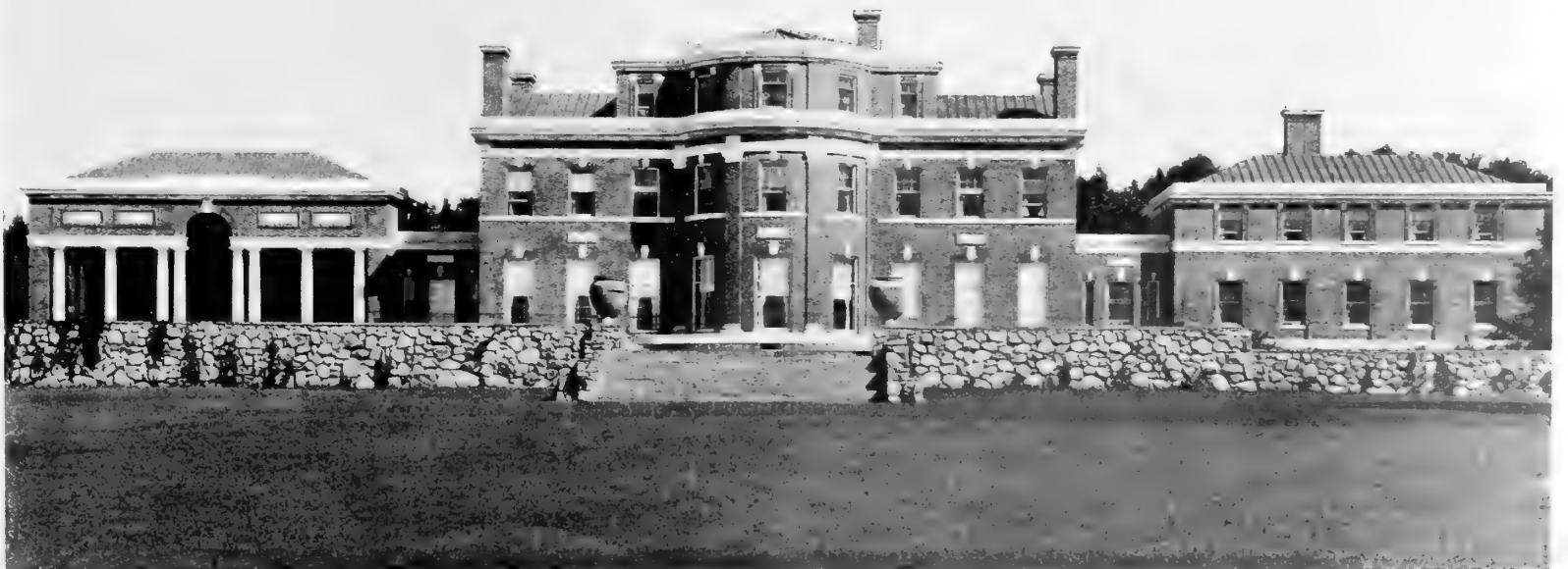
The Stately Water-front Shows the Three Great Divisions of the House, with the Portico to the Left
